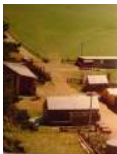
Farm sheds at Table Cape
